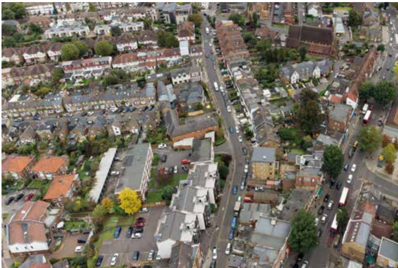
Image: Aerial view of Hanwell Town Centre.
