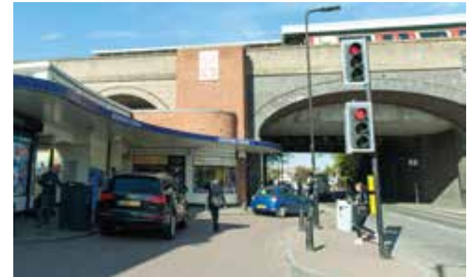
Image: Greenford Station, Oldfield Lane North.
