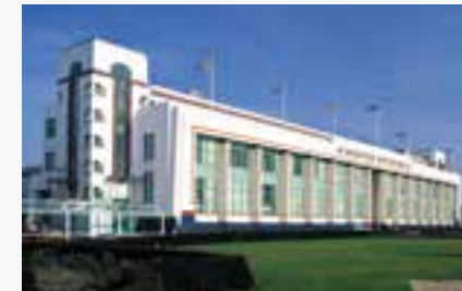
Image: Hoover building, Perivale.
