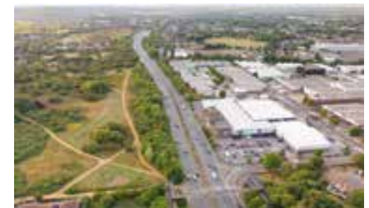
Image: Aerial view, A40 Road, Greenford towards Northolt.
