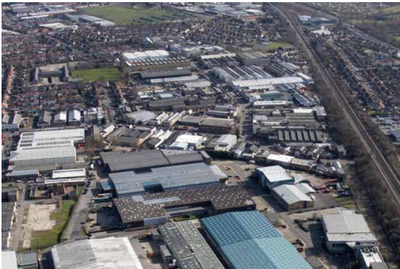
Image: Perivale industrial estate.
